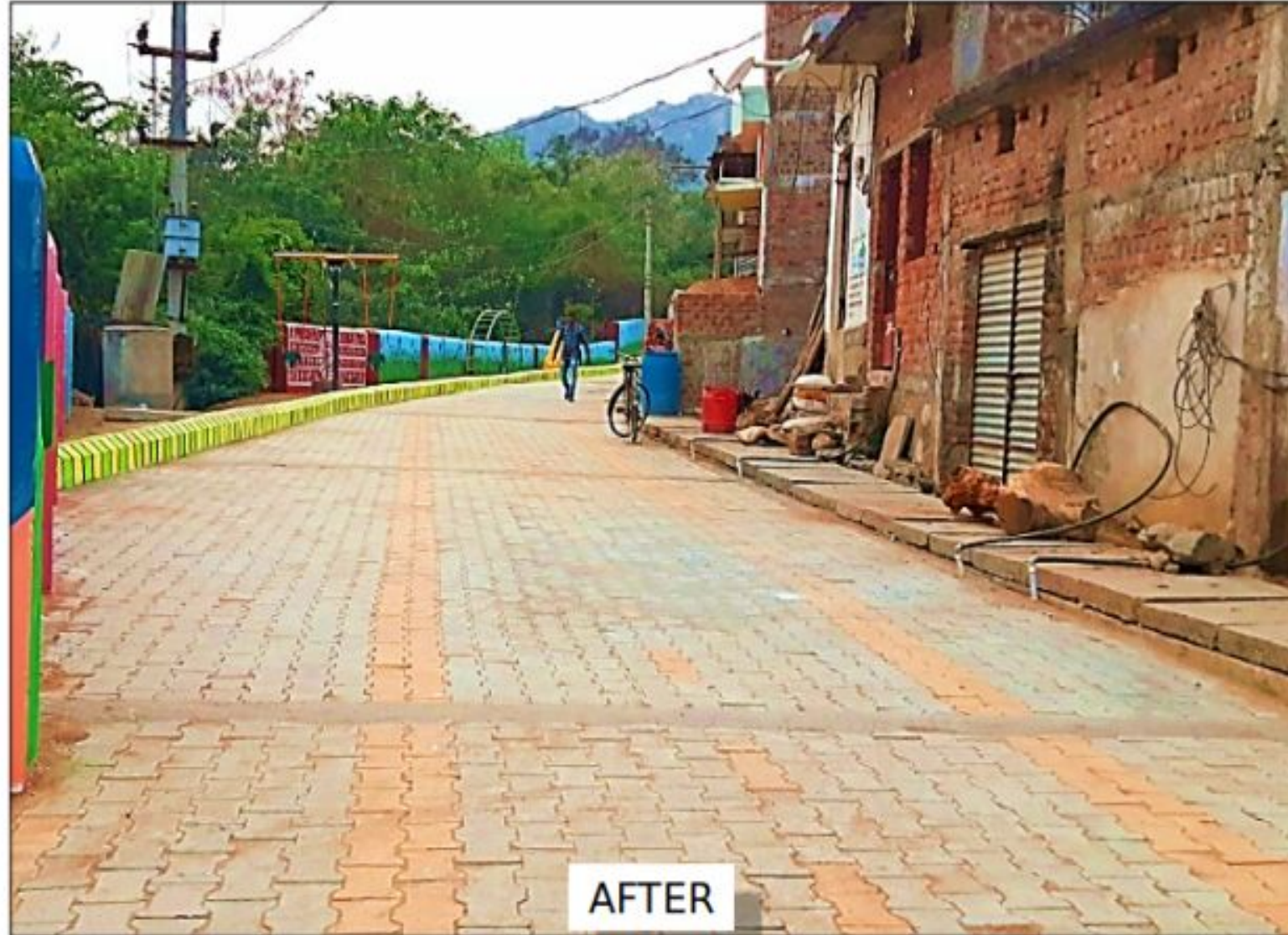
Paver Blocks laid for road development in slums of Hinjilicut
